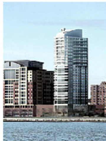
W Hotel in Hoboken upon completion.
